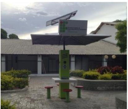
Figure 4- Photovoltaic system used for supling DC current. Source: Own autorship.
